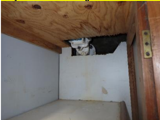
Grey Water OB discharge Valve Stbd of C.L (2CZ1)
