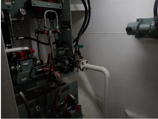
Omnipure OB Swing Check Valve
