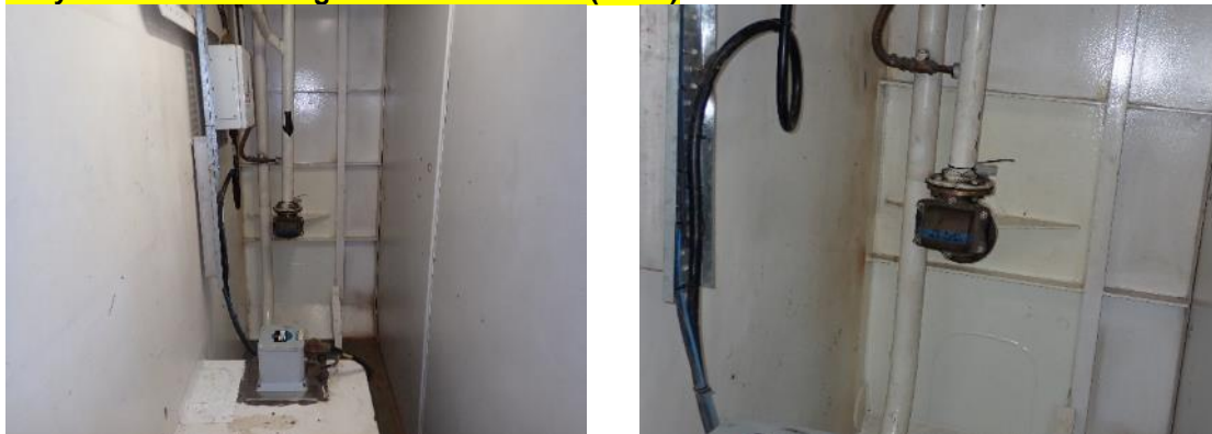
Sonar Cable Conduits Blanked & Sealed Stbd of C.L Fr.32 – Fr.33
