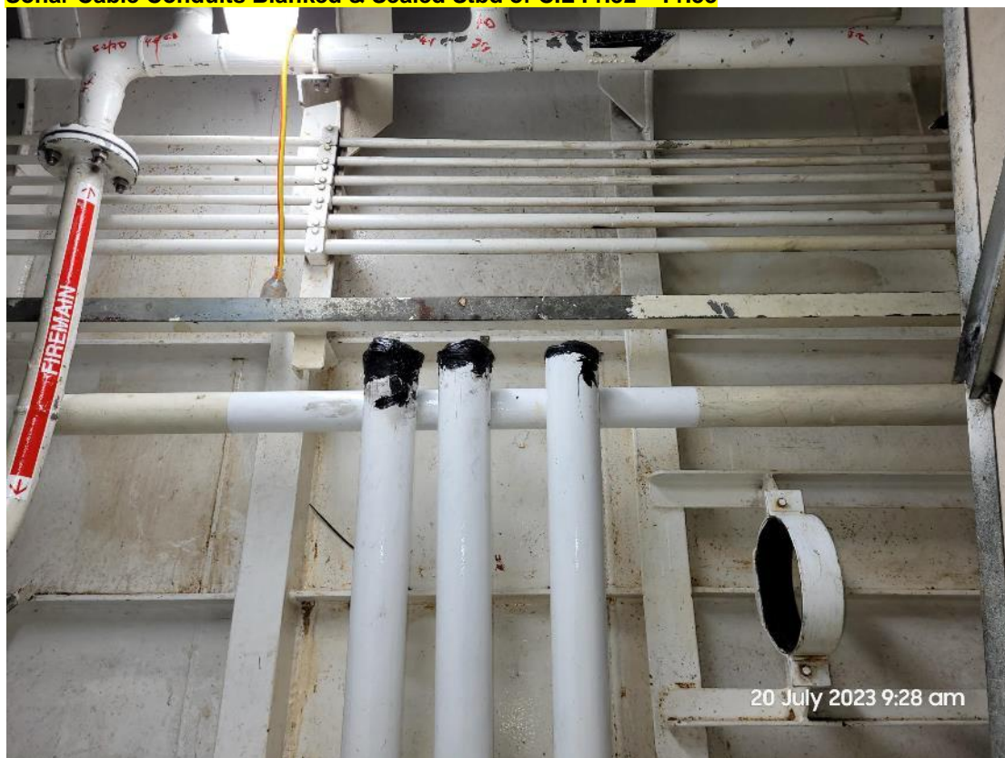
Sonar Cable Conduits Blanked & Sealed Stbd of C.L Fr.32 – Fr.33
